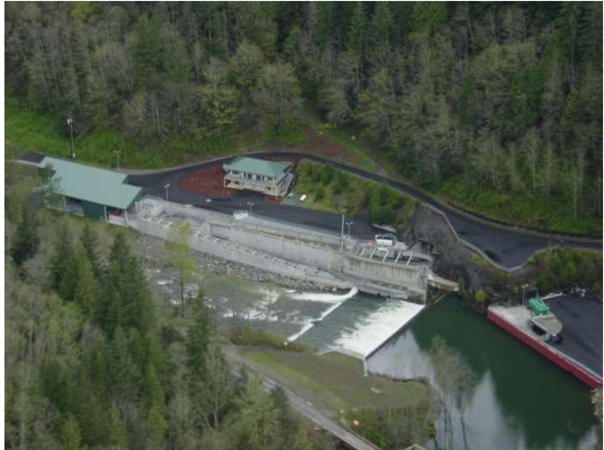
TACOMA WATER DIVERSION DAM AND INTAKE
