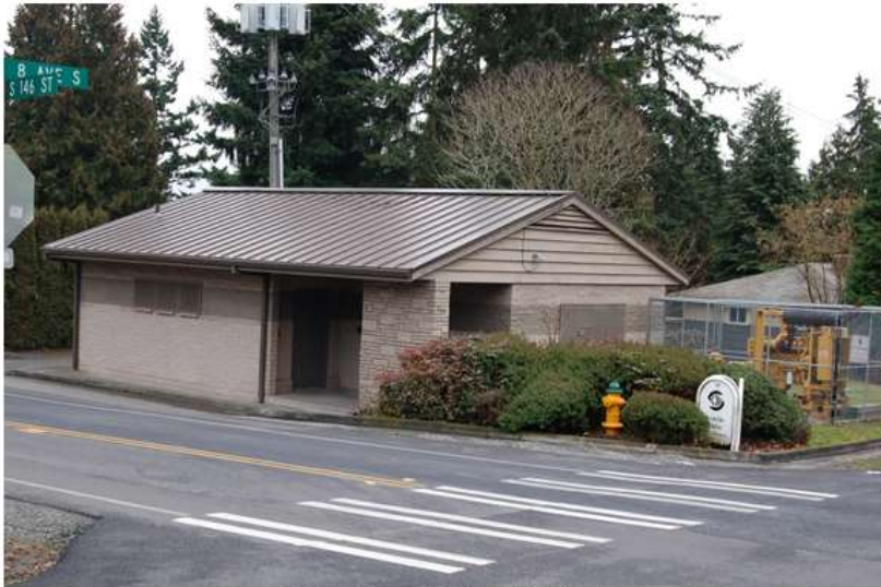
Burien Pump Station Site Photo
