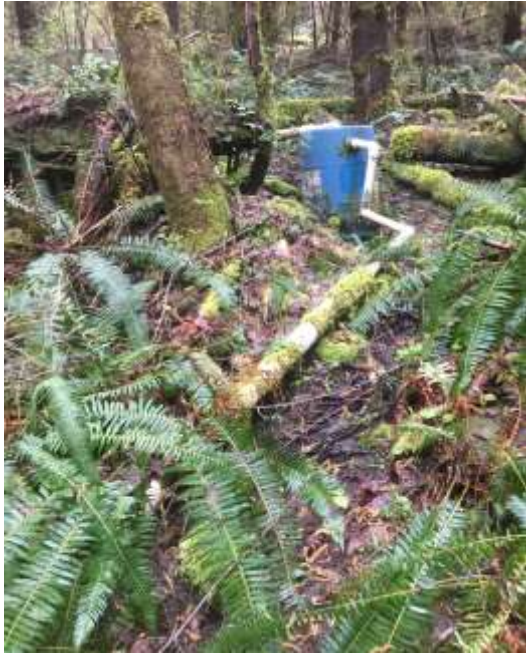
Barrel line settling basin (KISS)
