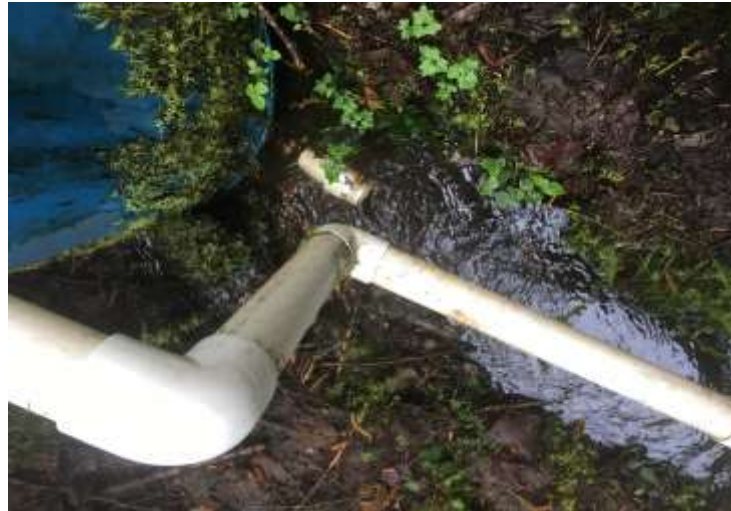
Barrel line bottom cap open during winter and closed during summer
