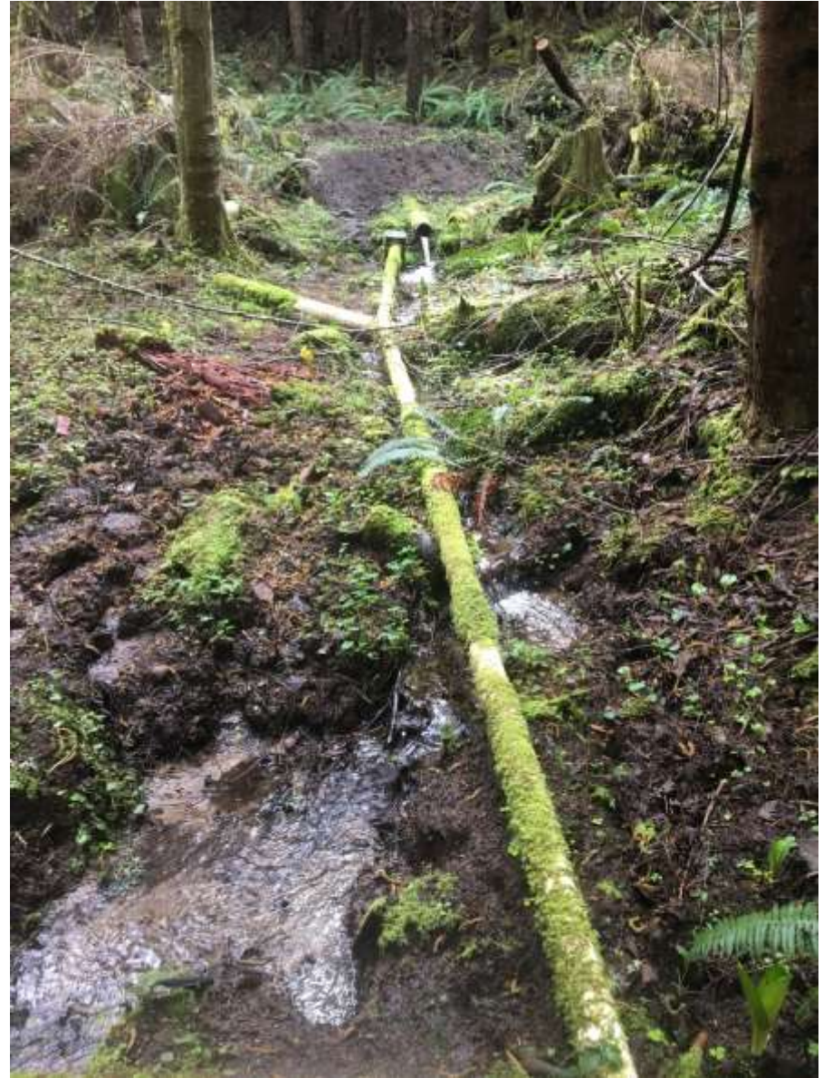
Water leaving the sediment basin, flowing into the catch bucket for the piping to distribution box.
