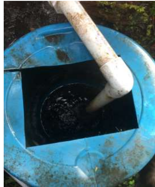
Overhead view of Barrel line, settles debris, reduce turbidity to reduce costs of chemicals for treatment.
