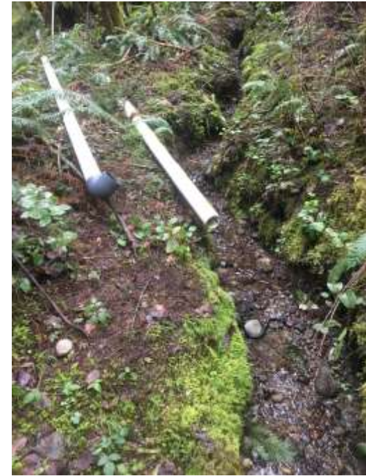
End of piping for #5 N.
