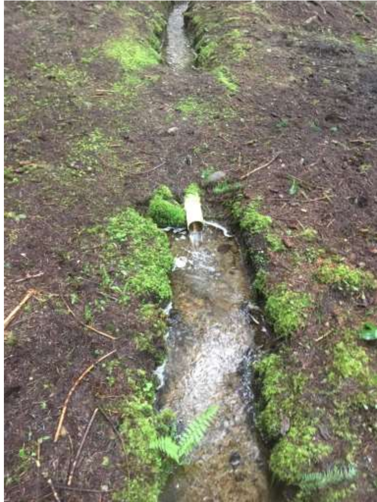
End of Orangeburg Line prior to piping into Little Camp Creek
