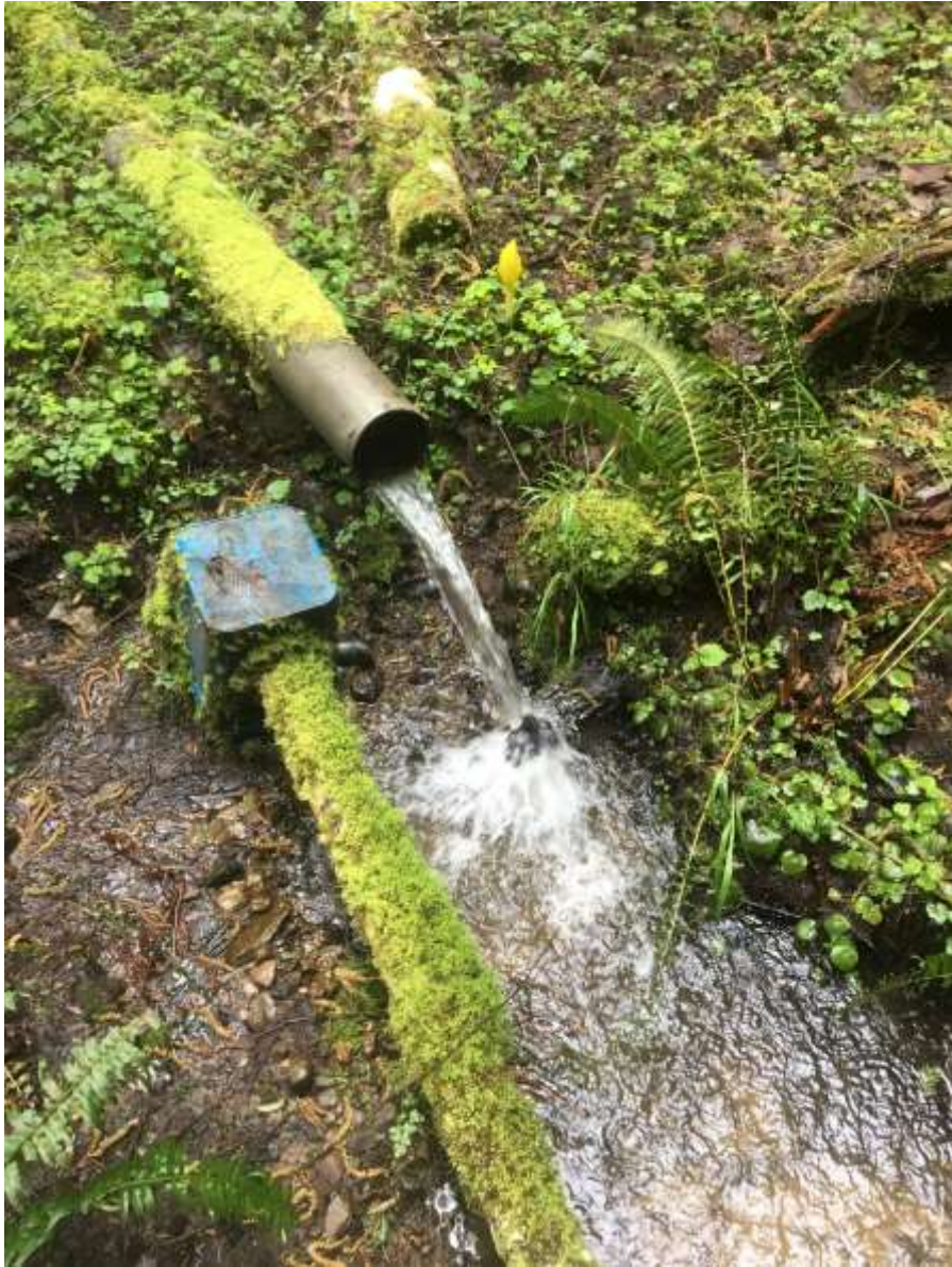
Water leaving the sediment basin, flowing into the catch bucket for the piping to distribution box.
