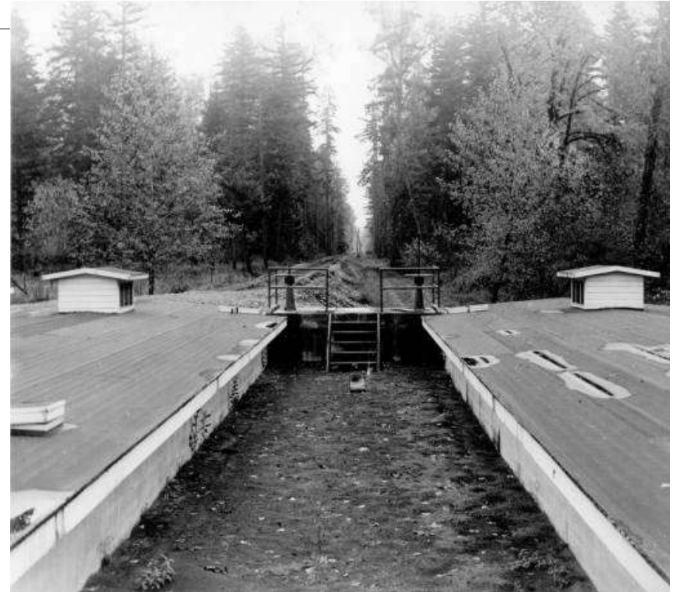
Sand screen facility looking upstream on Geren Island, 1956. (Oregon State Archives, Ben Maxwell Collection, 1075)
