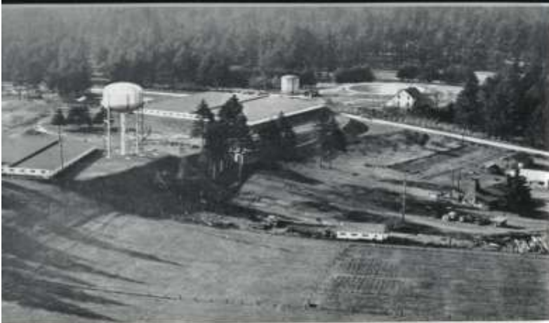
Station No. 1, reservoirs and tank on hill; well and meter-tap on right.
