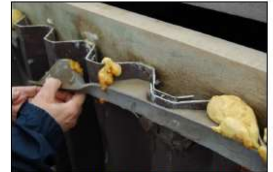
Foam Eave Filler at North Elevation Flashing
