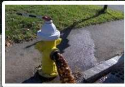
System Flushing
