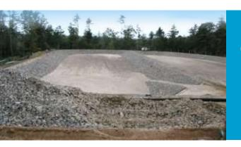
Class A recycled water pumped to infiltration site and discharged to infiltration basins (summer only)
