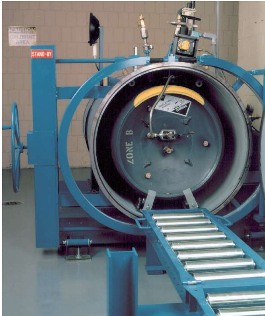
Typical Chlorine Containment Systems for Ton Container
