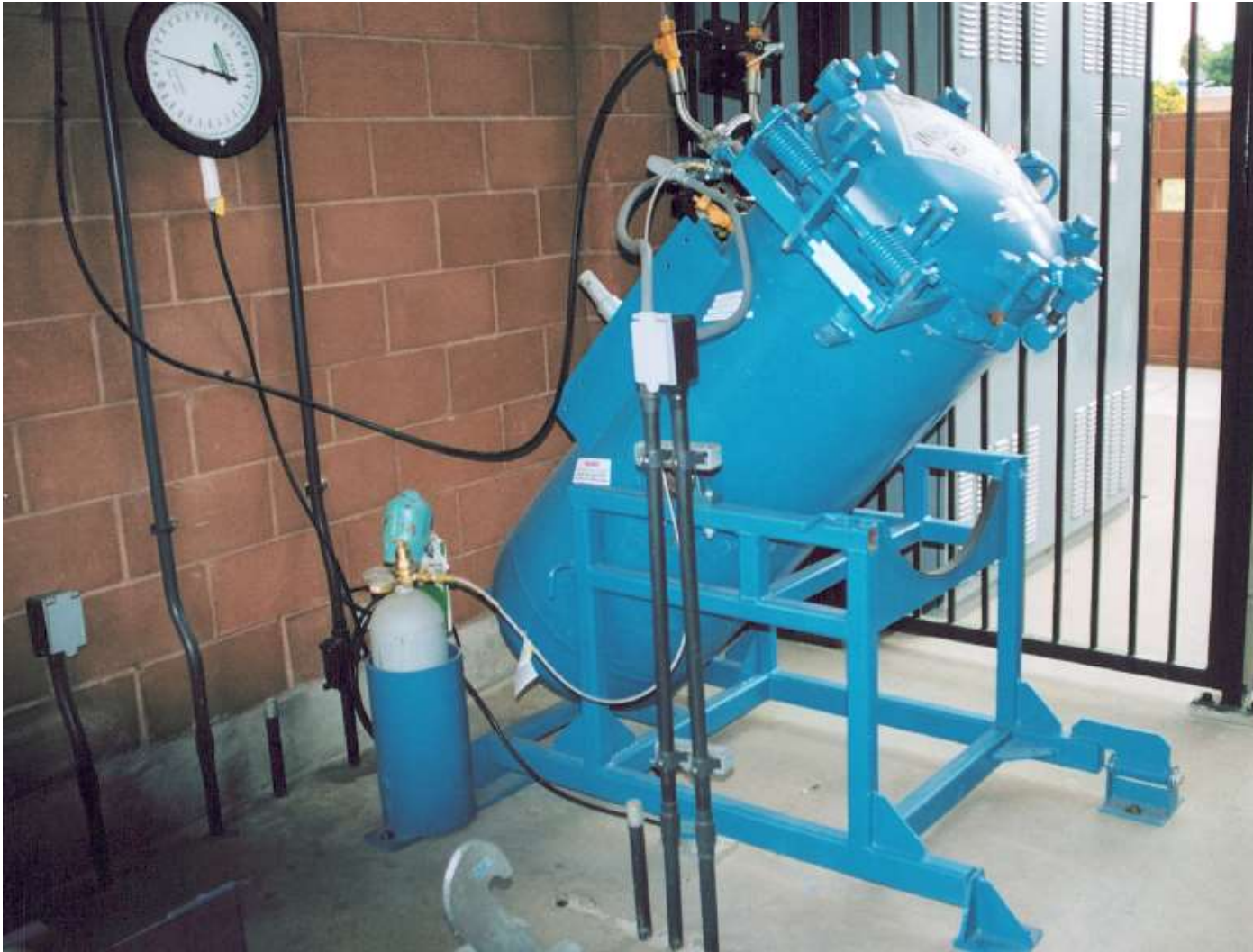
Typical 150 Lb Cylinder Containment System
