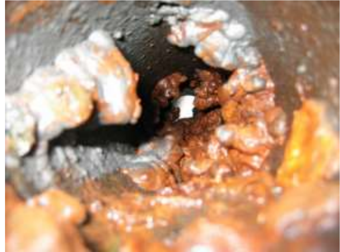
4-inch Unlined Cast Iron Main
