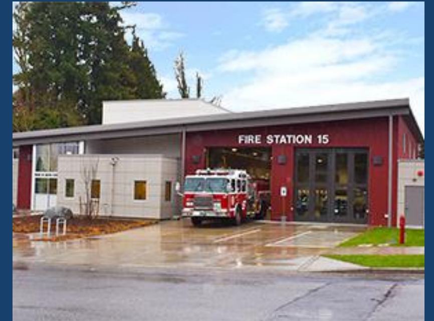
Leverage Fire Station Construction
