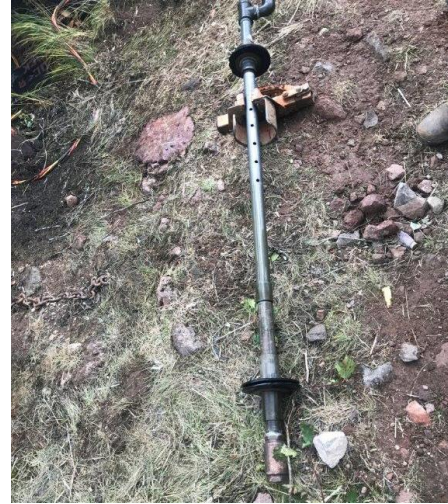
Developed with air + Airlift debris from well
