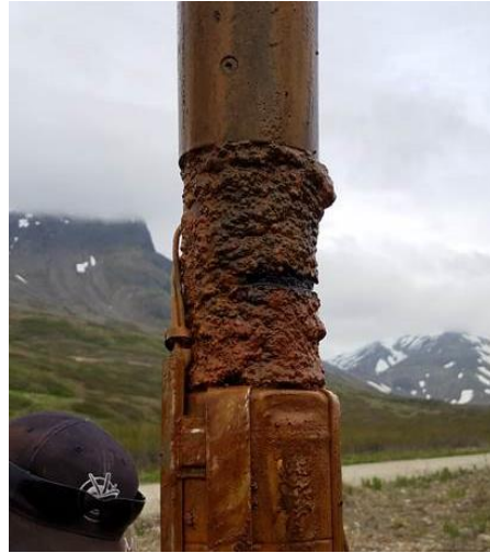
Visual Inspection – Inspection of column pipe and pumps
