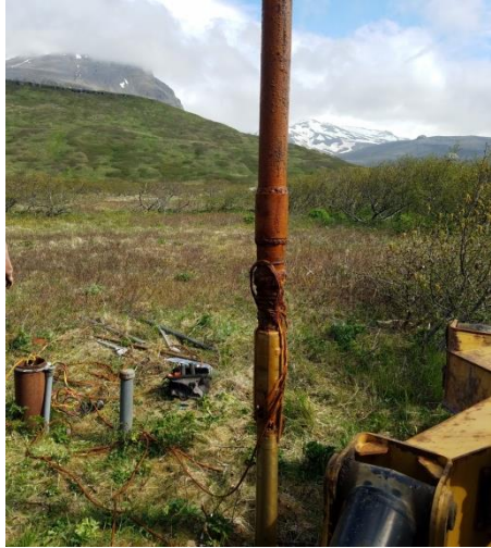
Removal of Pump and Pipe
