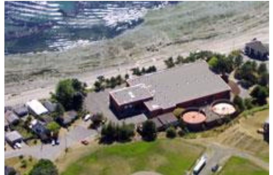
KC ALKI CSO TREATMENT FACILITY
