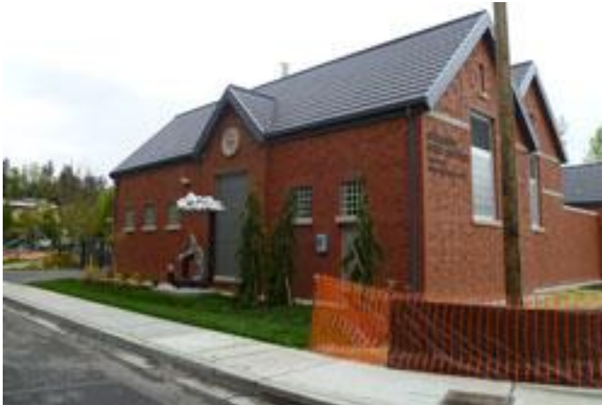
KC BELLEVUE PUMP STATION
