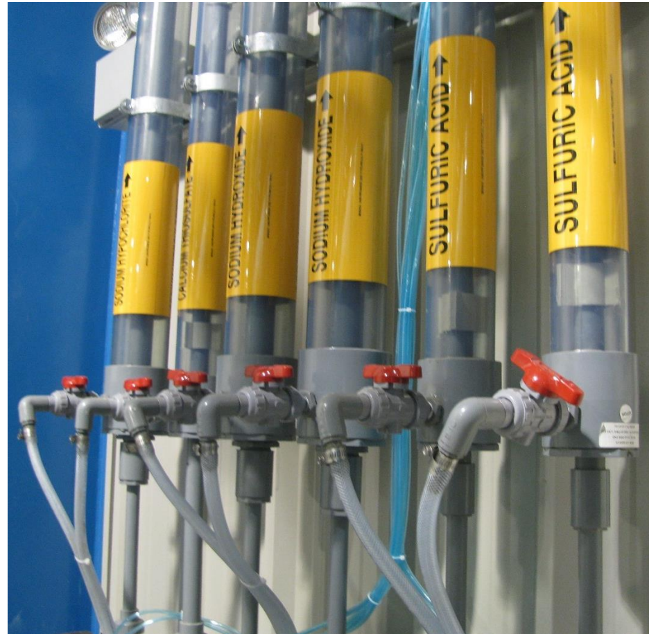
Single-walled pipe with transparent shell
