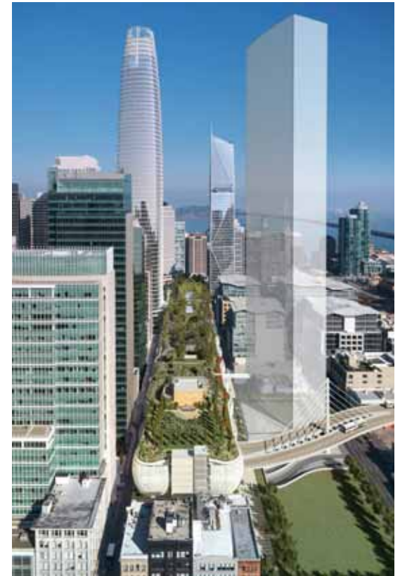
San Francisco Transbay Terminal
