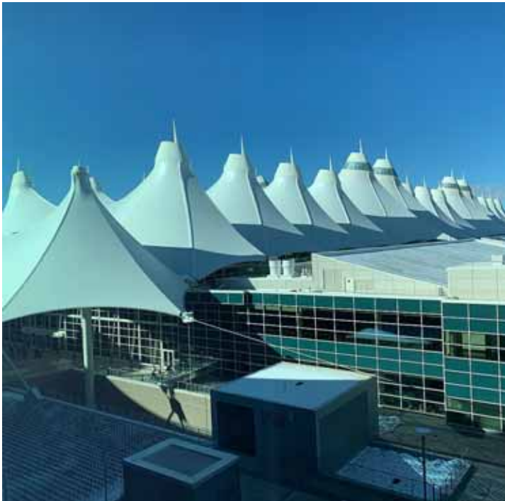
Denver International Airport - $2 billion over budget, 16 months behind schedule. Actual traffic 55% of forecast in opening year
