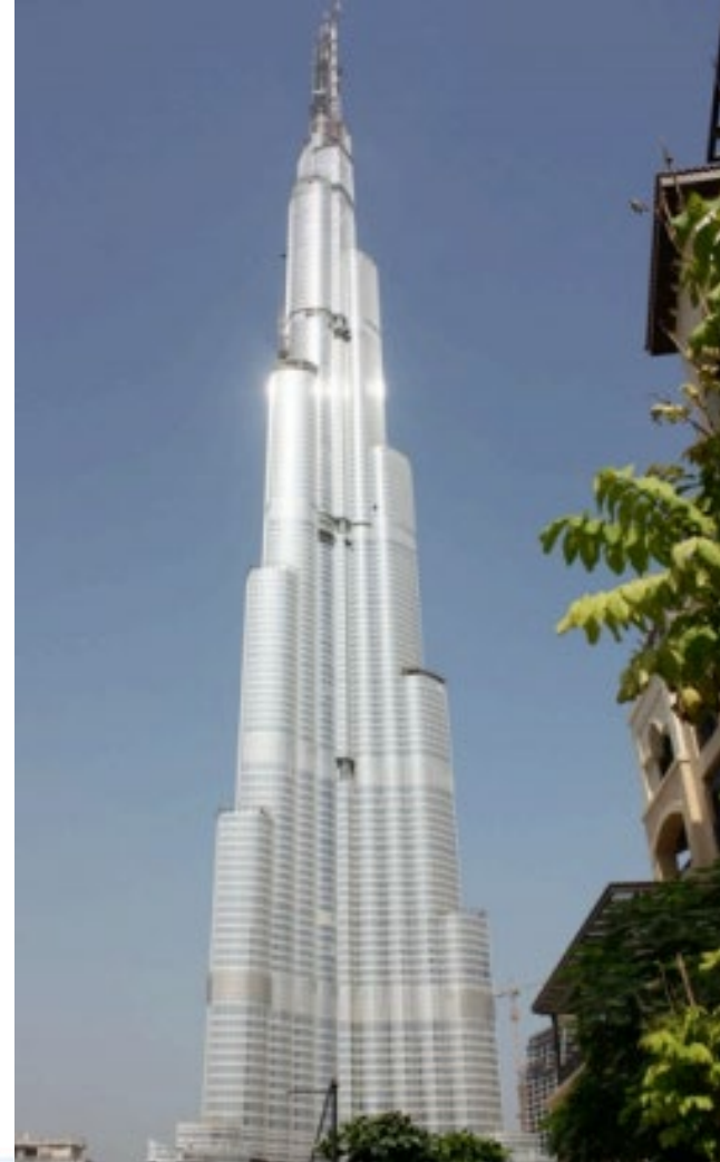
Burj Khalifa Dubai, U.A.E. (Tallest Building in the World)
