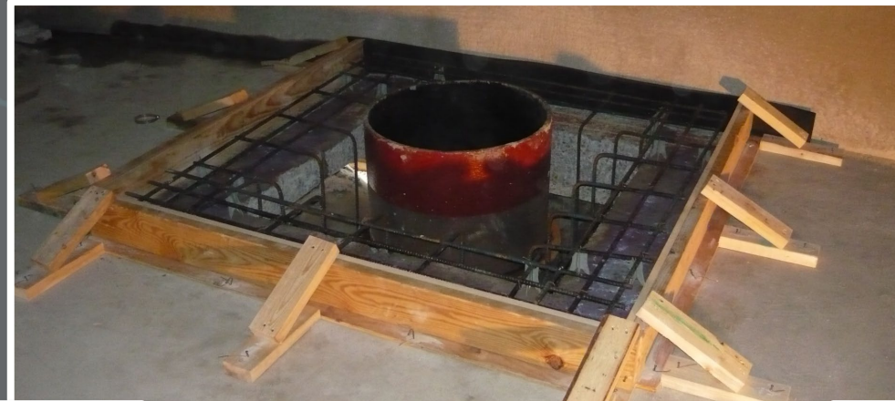
Forming New Penetration
