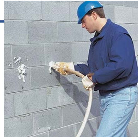
Florida Energy Solutions
