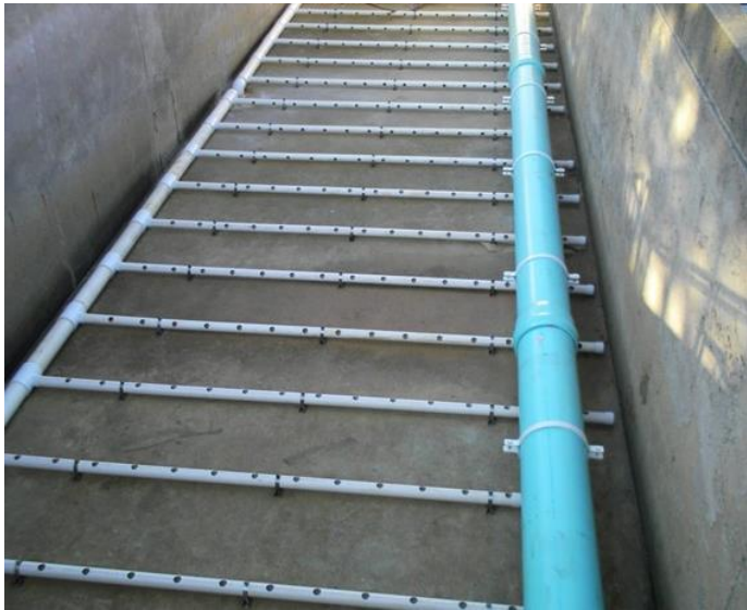
Fixed Grid Orifice
