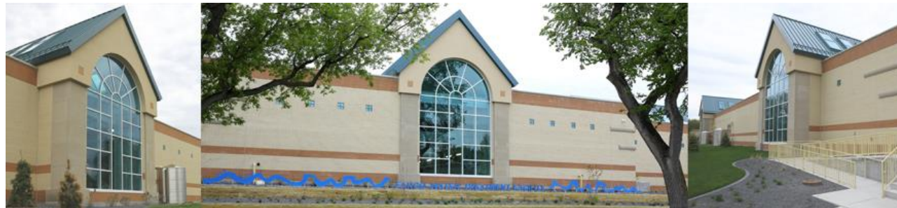
Fargo Water Treatment Facilities Fargo, ND
