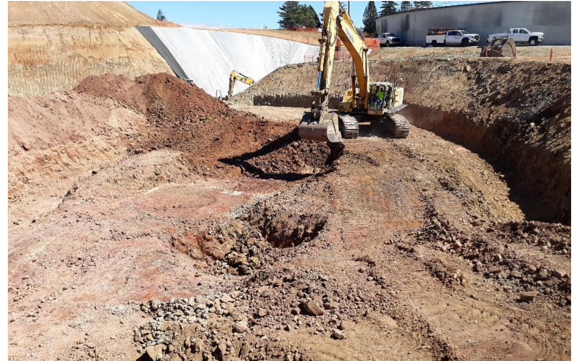
Overexcavation of decomposed basalt. Area backfilled with 500 psi lean mix
