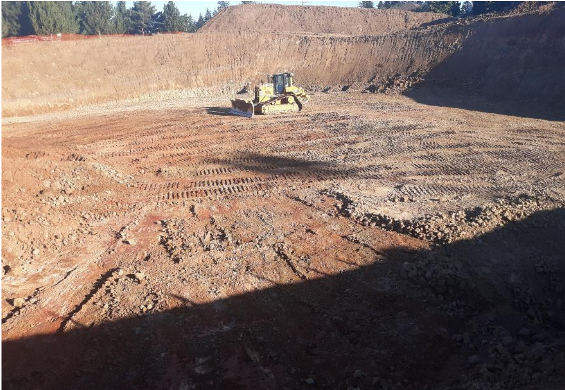
Subgrade typical R1 (very soft) or harder basalt
