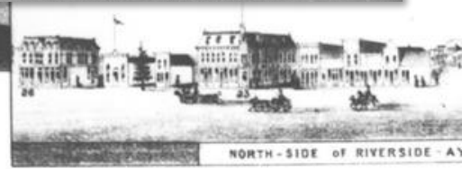
NORTH-SIDE OF RIVERSIDE-AVE.
