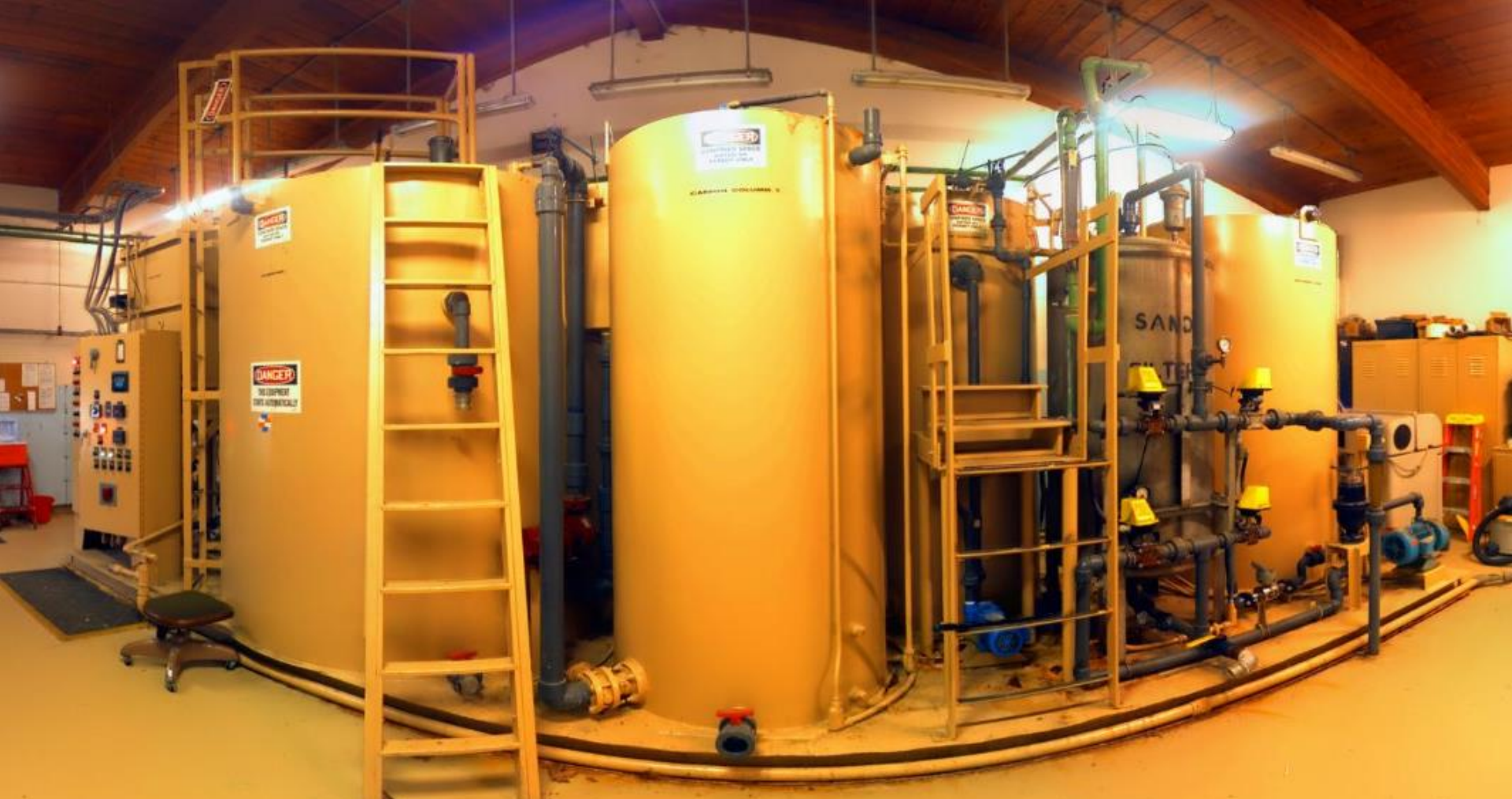
Constructed 1974, Skid replaced in 1980s, Rehab'ed in 2000
