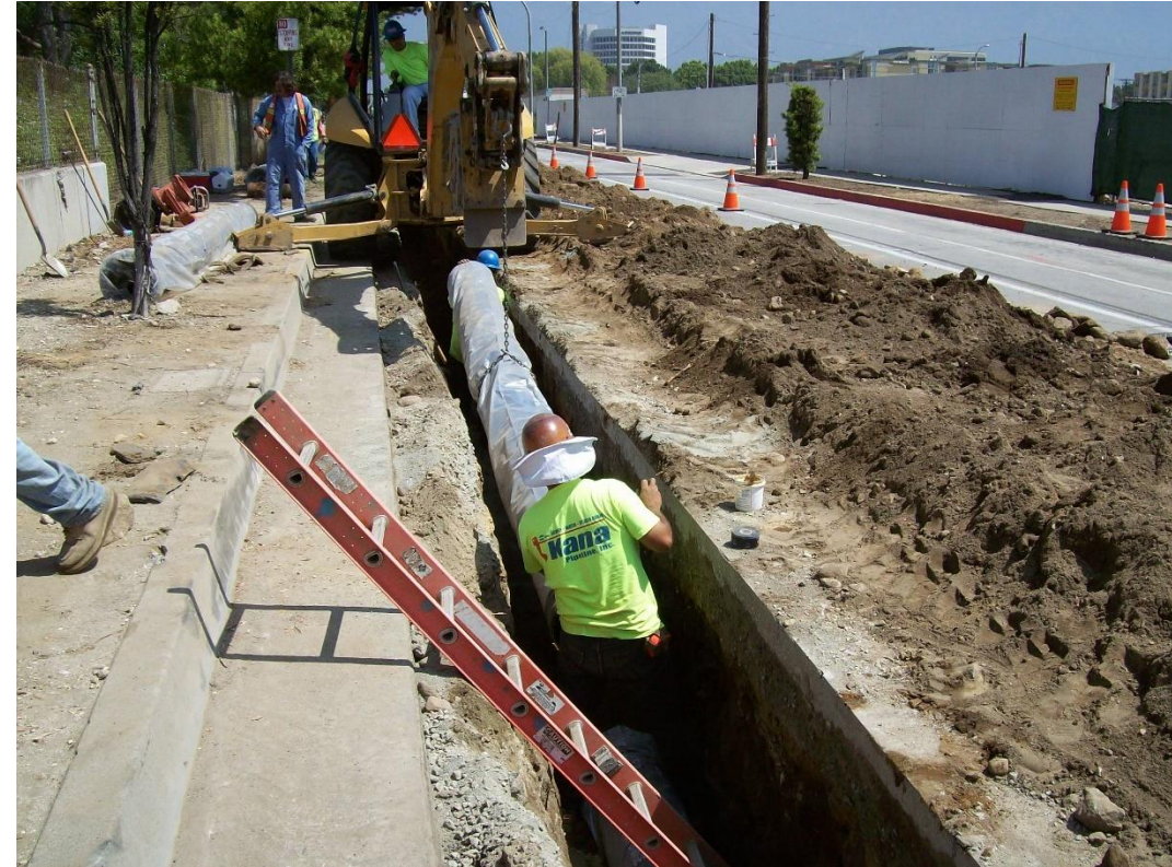
Photo from Kana Pipeline, Inc.
