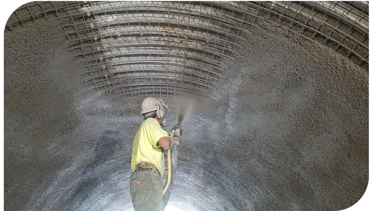
Example Pipe Lining Shotcrete Application
