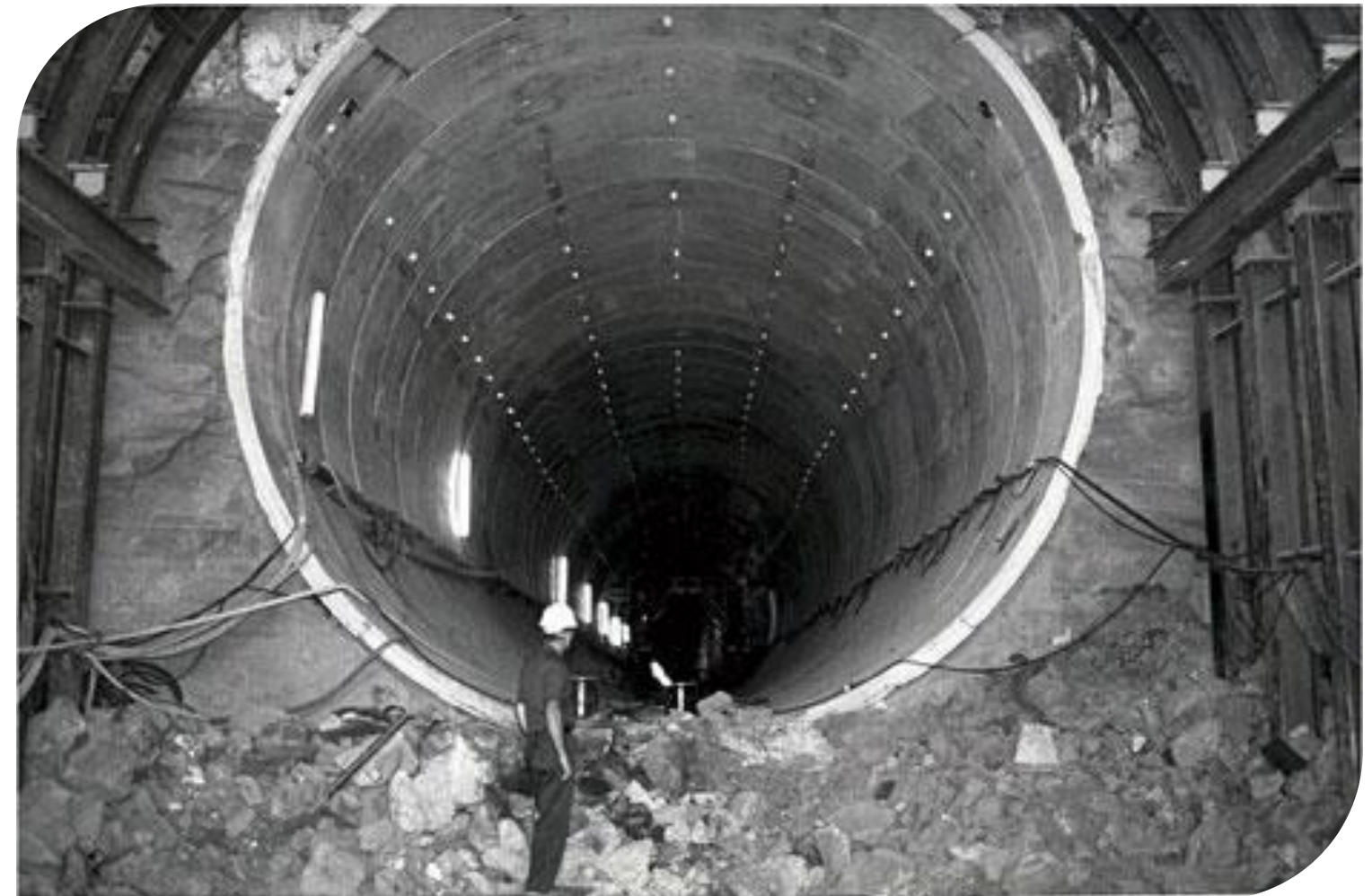
CAP Tunnel at Lake Havasu
