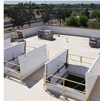
Elevated entrances, bridge cranes and access hatches
