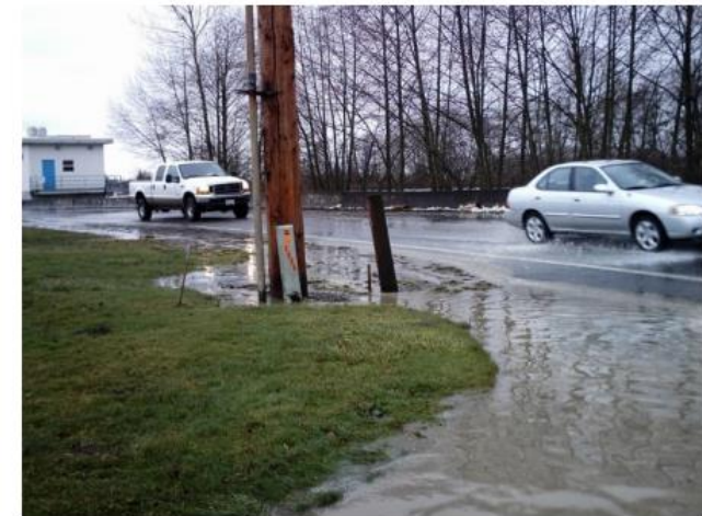
2009 storm event at WTP1 site
