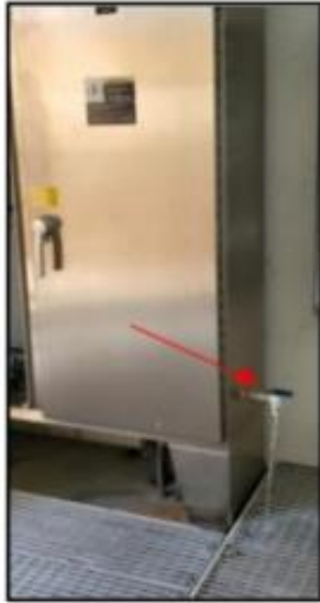
Combined Filter Effluent (CFE)
