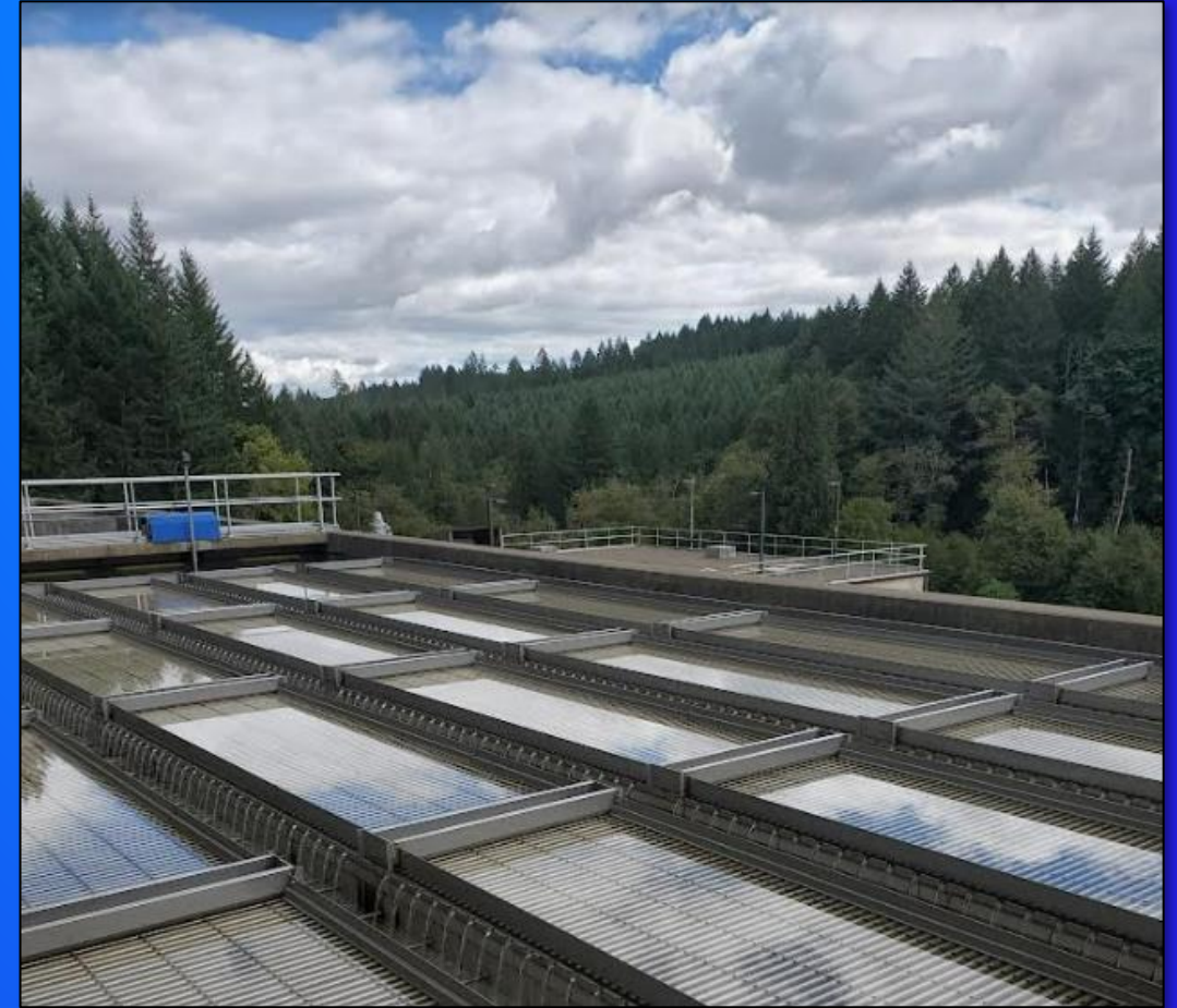
Norman Scott WTP, McMinnville
