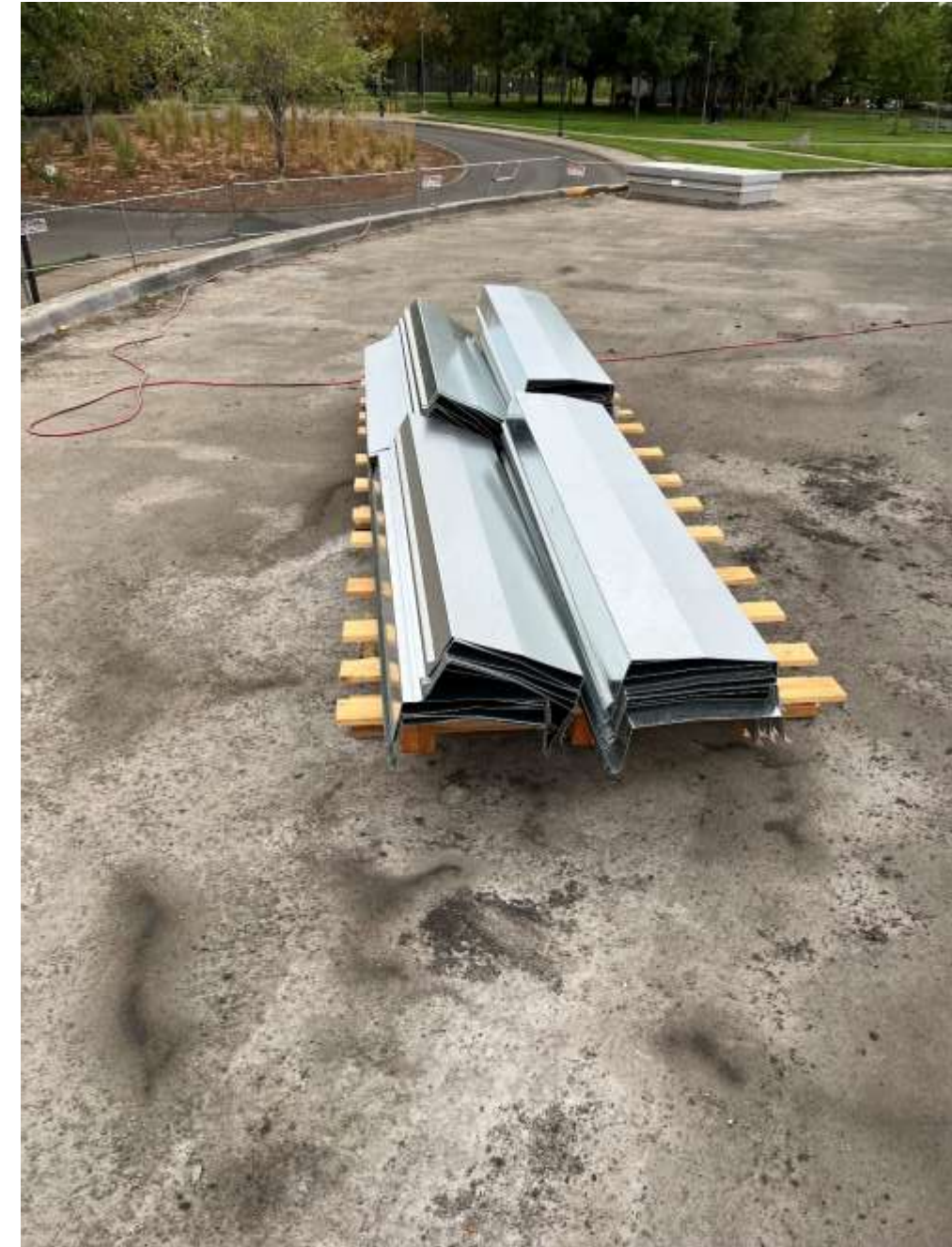
Top of wall flashing
