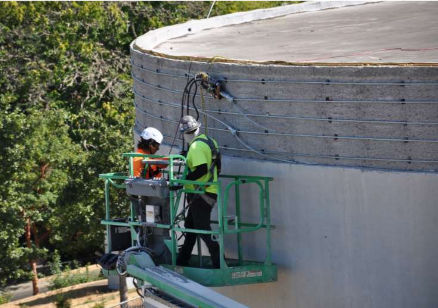
Dog bones installed at 4 locations
