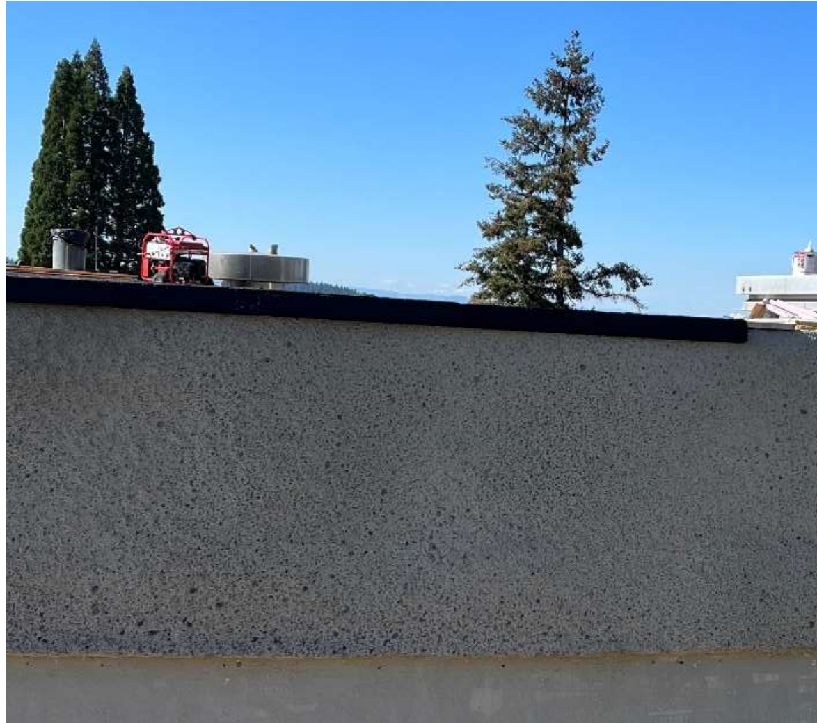
Foam filler at outside edge of wall
