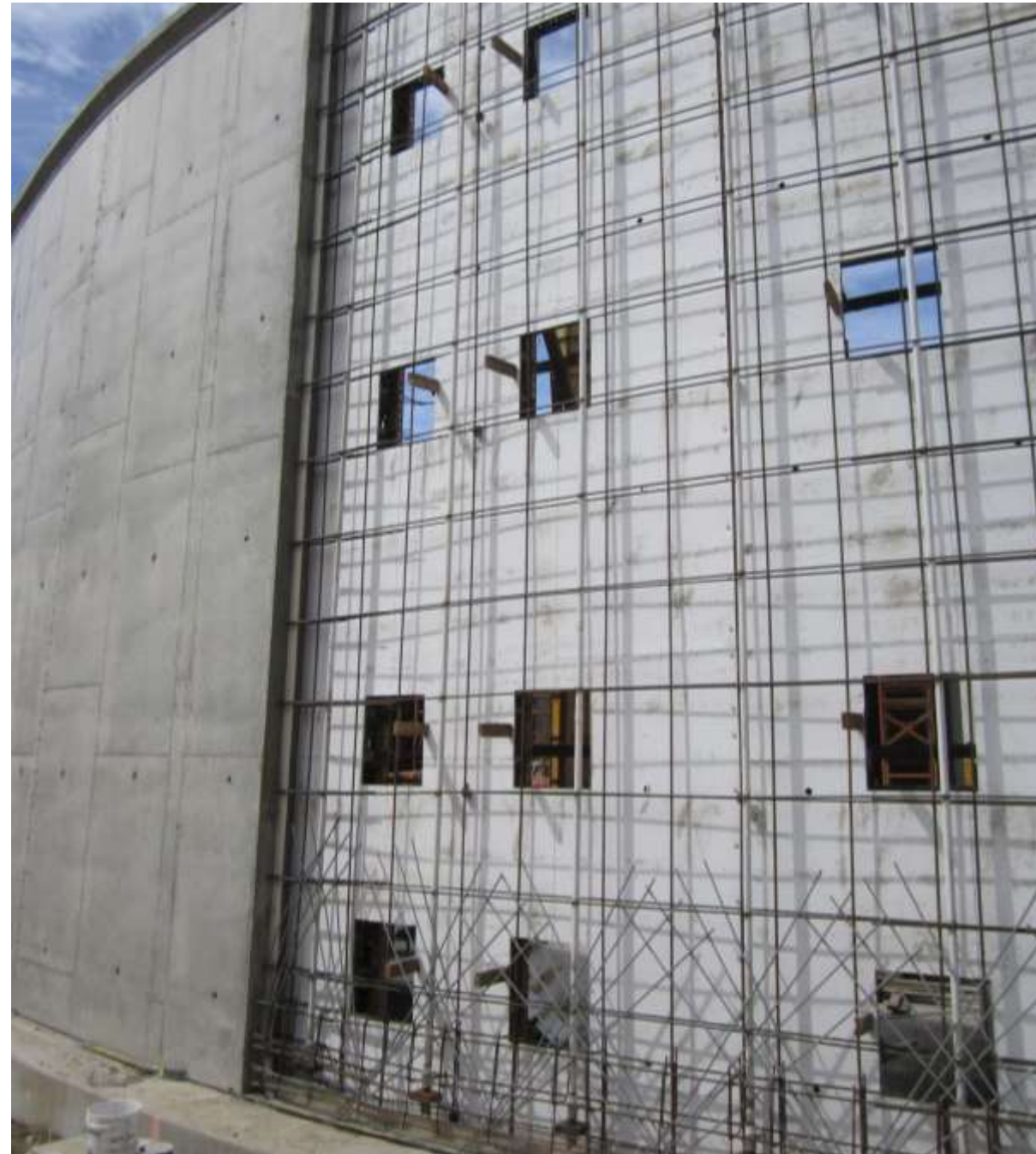
Typical Type I Wall Construction
