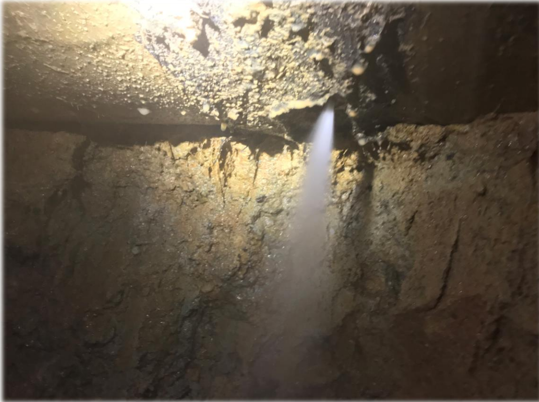
Pin-hole leak
