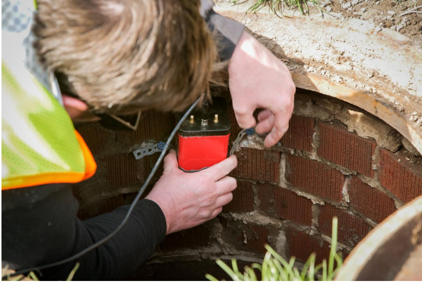
Electronic module typically mounted to the side of the chamber
