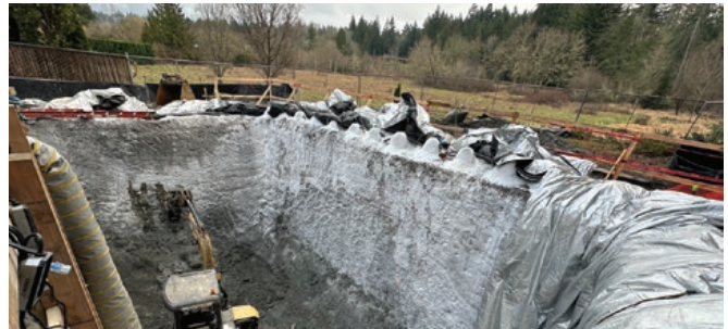
Figure 2: Shoring Method using SoilFreeze
